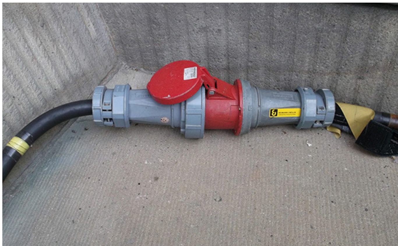
Figure 7: Notice the color coding (adherent to IEC 60309) of this high-power cable connector. (Image source: Railway Tech )
